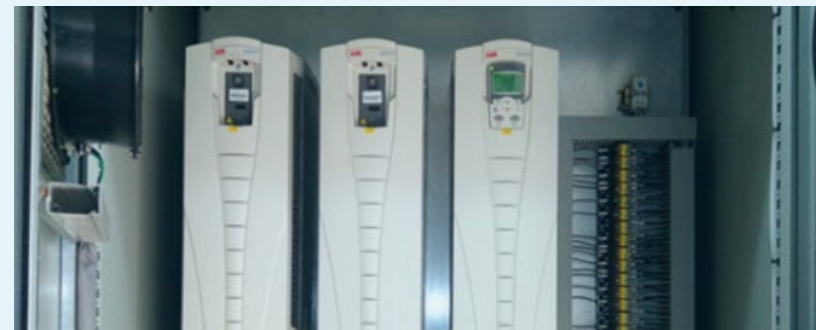
Adopting Variable Frequency Control for Facilities
