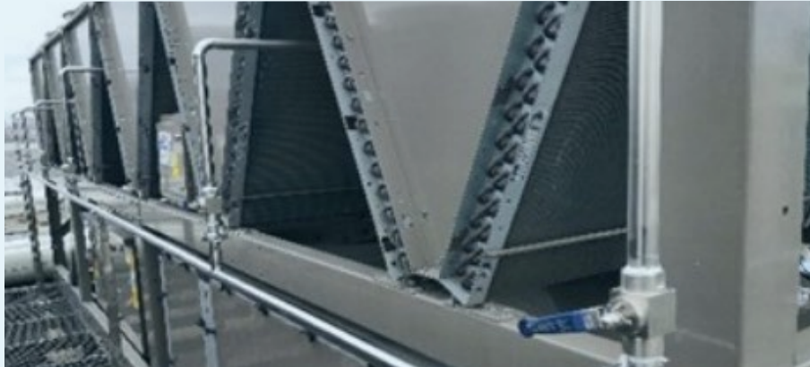
Transformation of the Fin-shaped Air-cooled Heat Pump Spray Cooling Pipes
