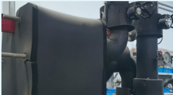
Heat Recovery of Steamed Condensate Water
